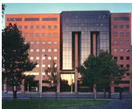
American Landmark Properties One Park Place, Syracuse, NY, achieved LEED-EB Silver Certification.
