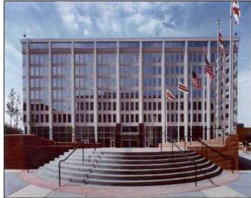
The Union Square Properties in Washington, DC earned LEED-EB O+M Silver Certification. From top: the 899 and 999 N. Capitol Street NE buildings.
