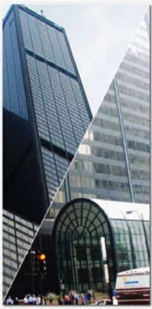
Willis Tower, Chicago, IL - location of live training in September.
